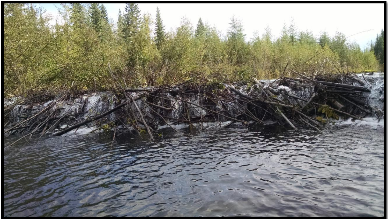
Dam 3 in August 2017
