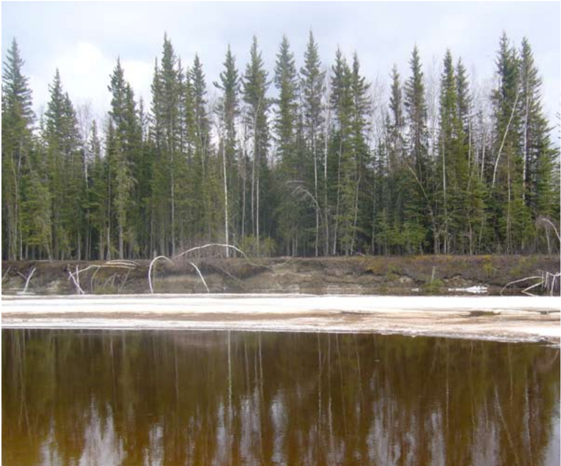
FIGURE 3. Chena River upstream of Nordale Road Bridge, showing shallow rooting of trees and vulnerability to erosion.
