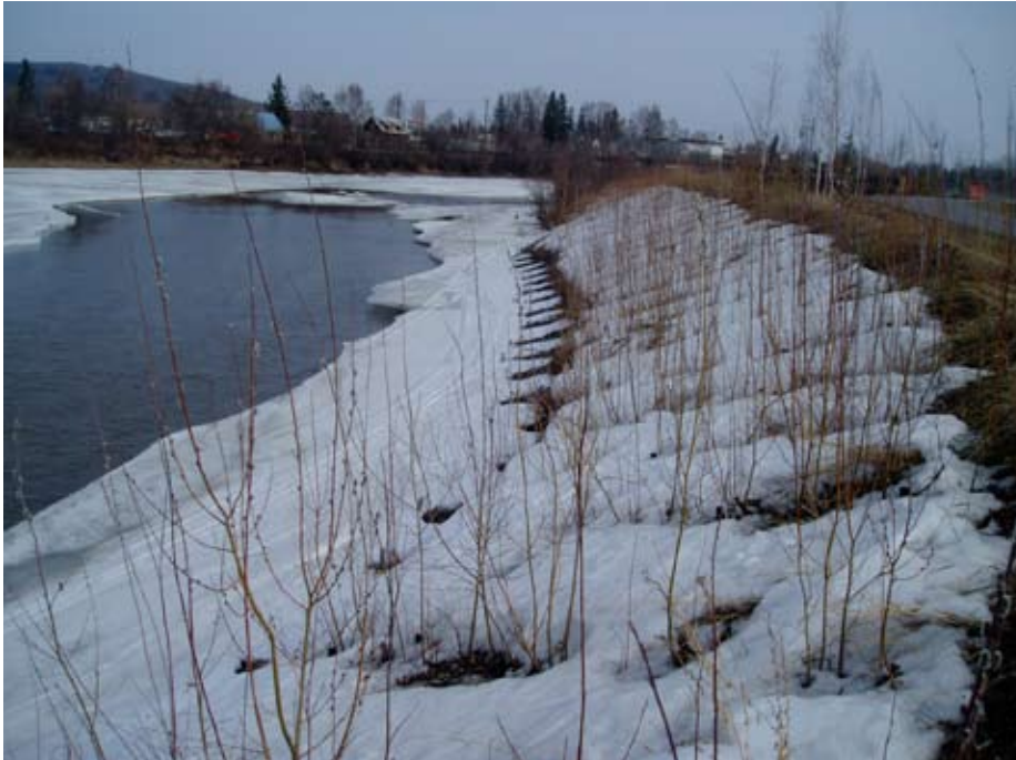
FIGURE 6. An example of a bioengineering project to stabilize the bank along the Chena River, near the Tanana Chiefs Conference building. This project involved covering riprap with soil and then placing willow bundles in diagonal rows on the bank.
