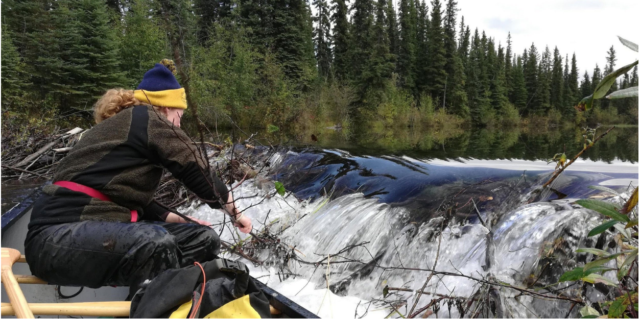
Site 1: TVWA contractor Jenna Jonas removes some of site 1 dam.
